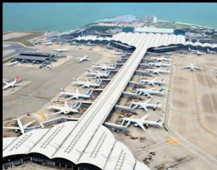
Hong Kong International Airport
