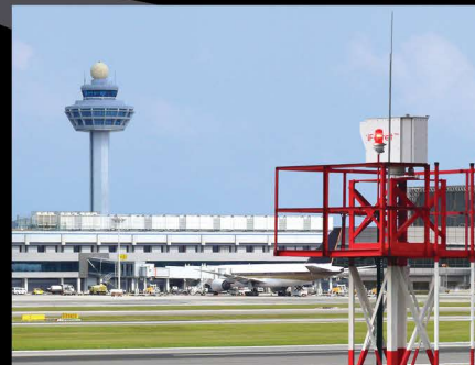
Changi International Airport (Singapore)
