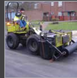
Installation performance per day - up to 20,000 m²/machine
