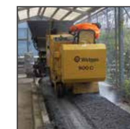
Milling the reinforced area
